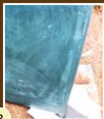
3 Painting 1st coat Using Sadocryl Auto paint
